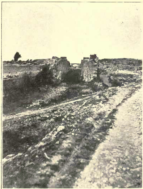
Part of the Useless Canal: shewing one of the Locks built of hewn limestone, intended to connect Lakes Mask and Corrib.
